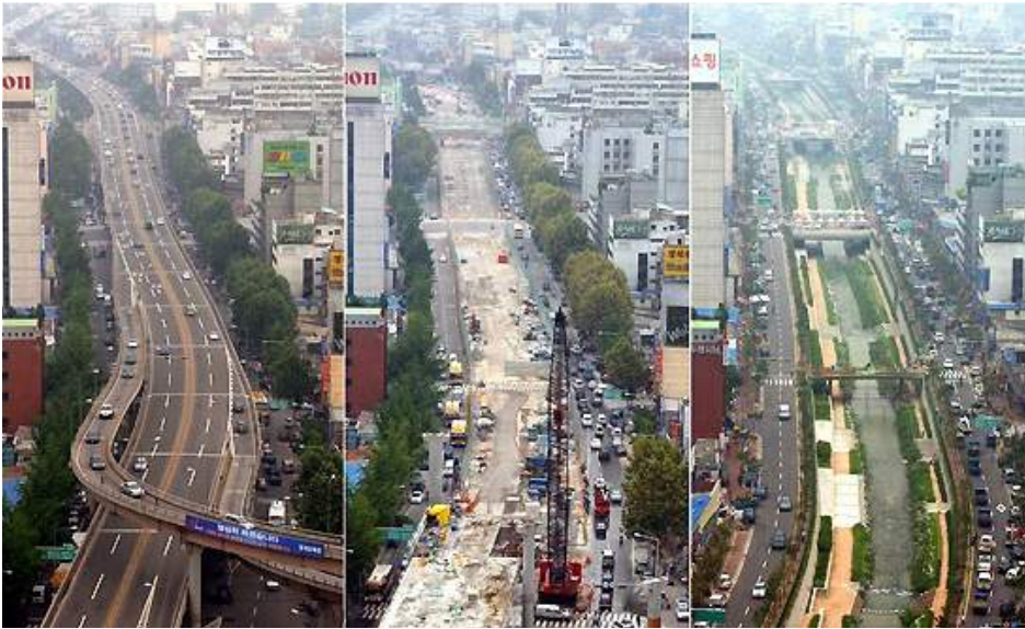
Fig 32: Process of Cheonggyecheon stream restoration (“Cheonggyecheon Stream The Restoration Project” n.d.)
