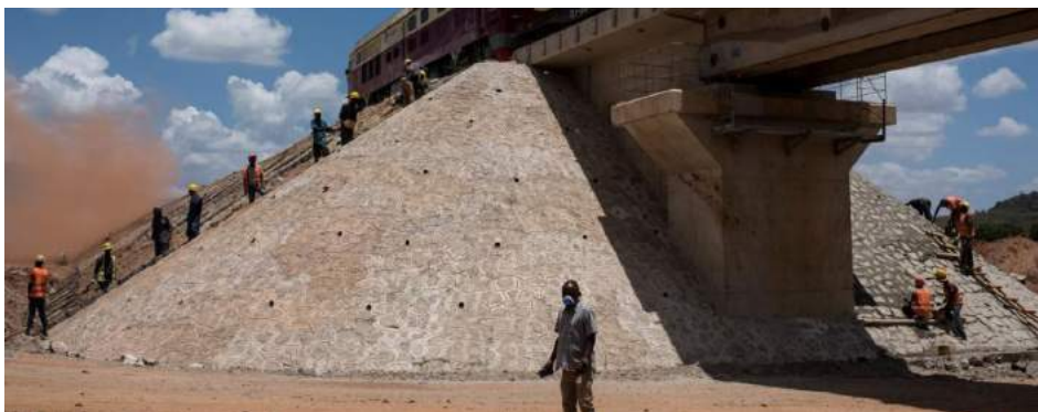
Fig 35: Embankments supporting the railway (NatGeoUK 2017)
